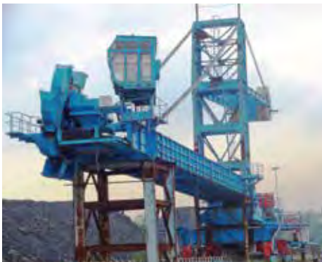
NALCO ANGUL - Coal Handling Plant for 2x120 MW
