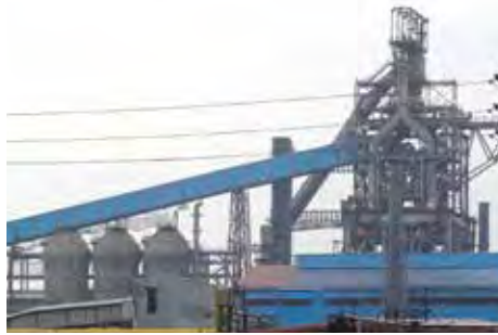
IISCO BURNPUR - Blast Furnace Changing Conveyer
