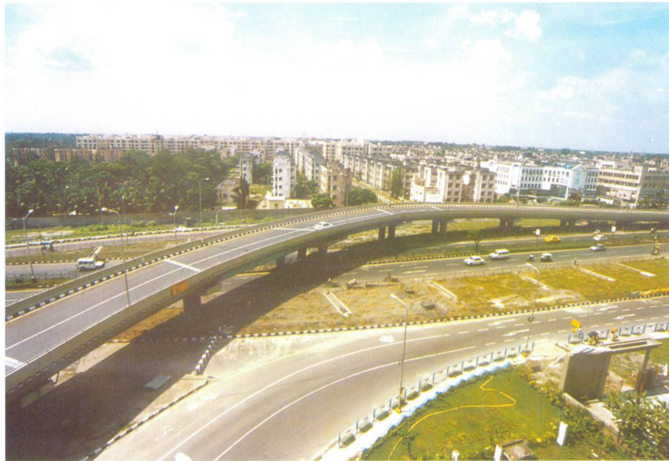
Birds-eye view of New Town Expressway
